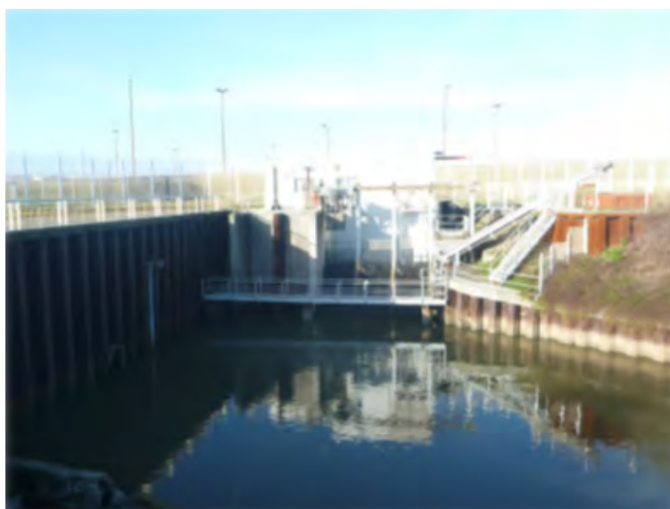
Figure 28 - Station de pompage de Marck - GCTM (source : Cerema)
